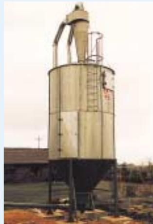
Silo with outfeeder and screw conveyor to wood waste burning system.
