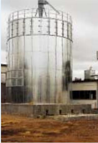
Insulated 396 m<sup>3</sup> silo with built-in wood waste burning system.
