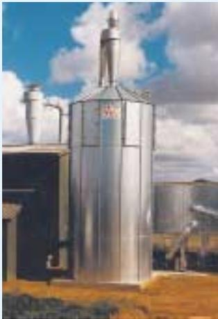
96 m<sup>3</sup> silo for wood waste burning system and emptying of suction car.
