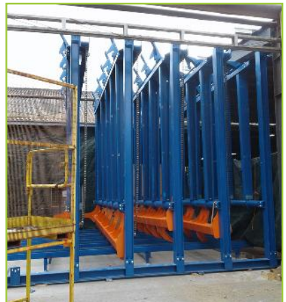
Installation of the box sorting line at James Davies Ltd.
